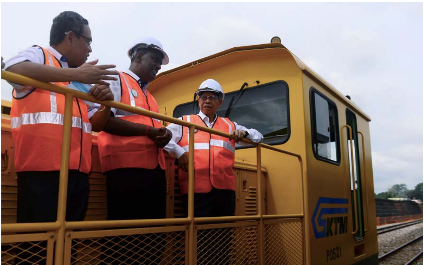
Datuk Seri Mustapa Mohamad is on a train with Datuk Jana Santhiran Muniayan while visiting the Gemas-Johor Bahru Electrified Double-Tracking Project site – Photo from fotoBERNAMA
