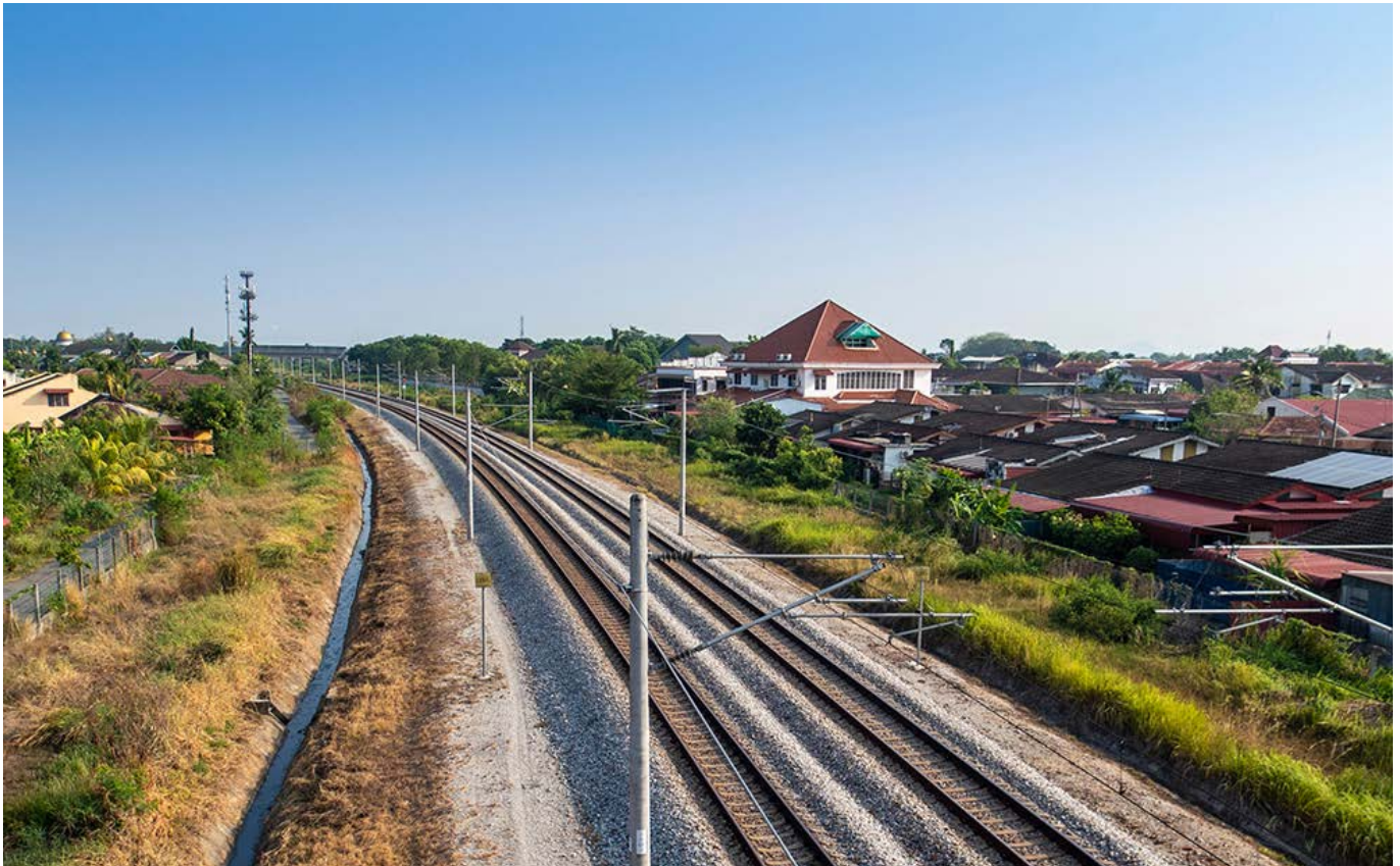
Birdseye view of the Gemas-Johor Bahru Electrified Double Track Project – Photo from Shutterstock
