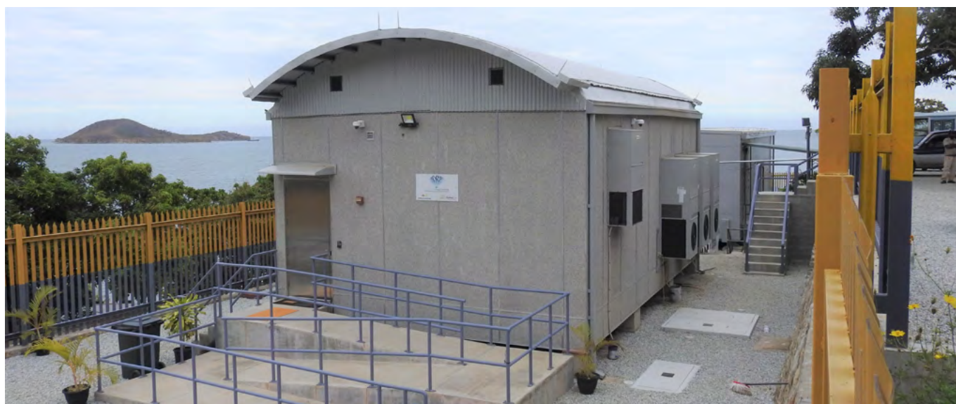
Figure 2. Coral Sea Cable Landing Station
